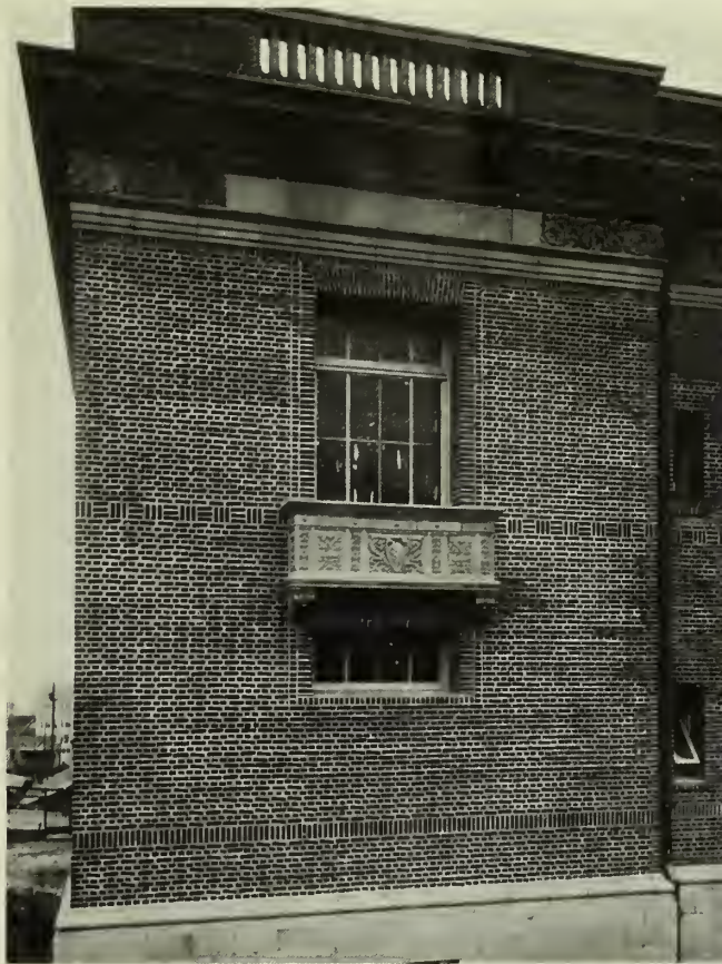
DETAIL, HANCOCK GRAMMAR SCHOOL. Newton J. Tharp and Loring P. Rixford, City Architects.
